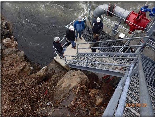
The entrance of the fishlift at river level below. The water enters the river below the person with the blue jacket. The large pipe delivers extra attraction water to the fishway.
