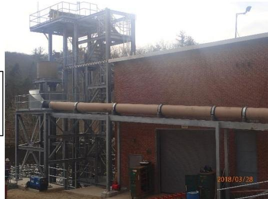
Right: The newly completed fishlift showing the long discharge pipe alongside the powerhouse.
